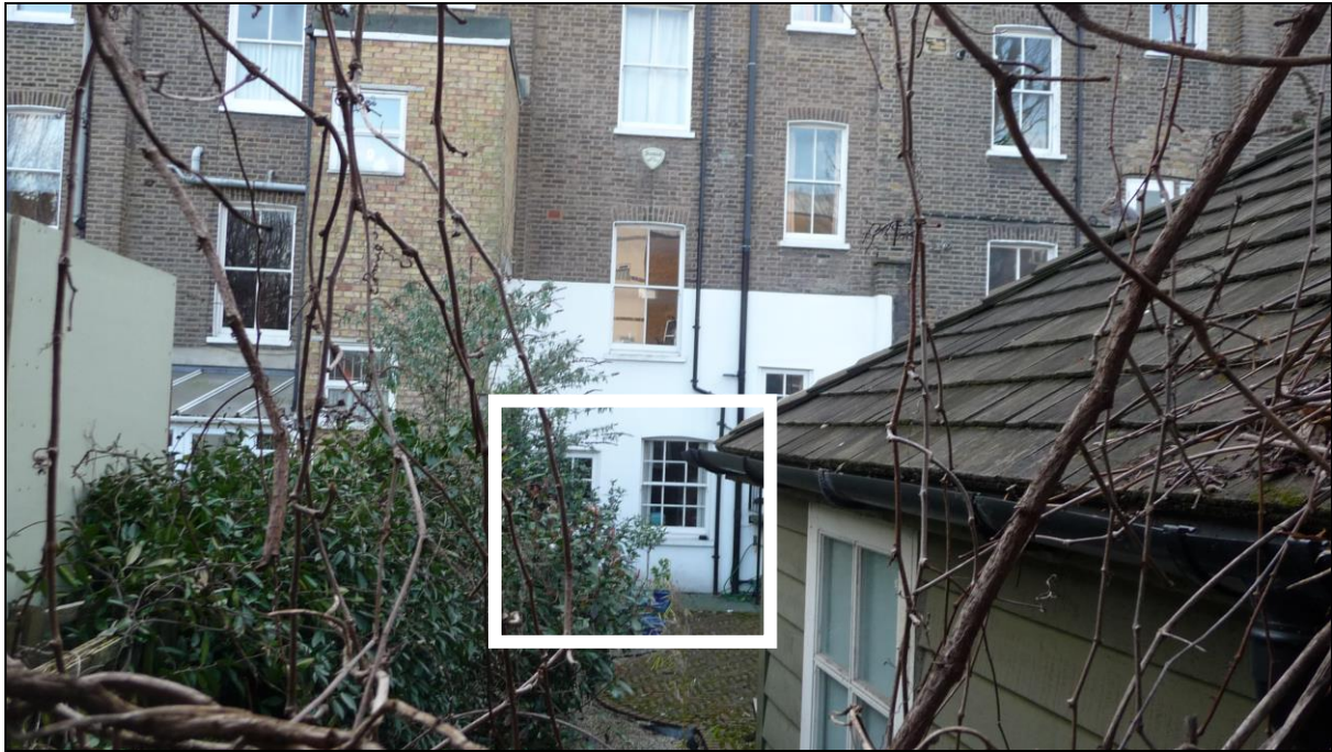
Fig. 28: Photo of the rear of No. 12 Packington Street. The room in question is lit by a window and glazed door (as outlined in white rectangle). Both window and door were taken into account in the daylight distribution analysis.
